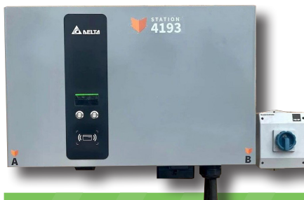
THE INSTALL: DELTA DC WALLBOX CHARGER
