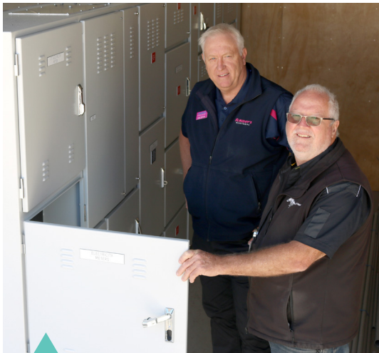
THE INSTALL: 800 AMP SWITCHBOARD UPGRADE & 440KVA GENERATOR INSTALL
