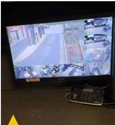
THE INSTALL: CCTV UPGRADES ACROSS 3 STORES
