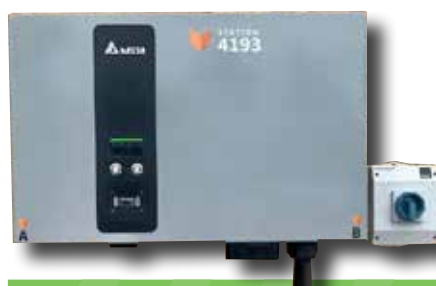
THE INSTALL: DELTA DC WALLBOX CHARGER
