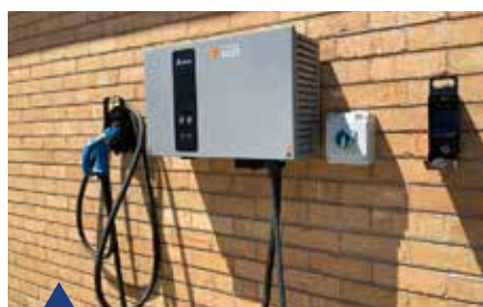
THE INSTALL: DELTA DC WALLBOX CHARGER
